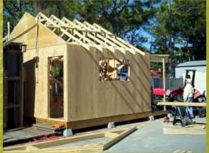
Officially UNDER CONSTRUCTION!!
